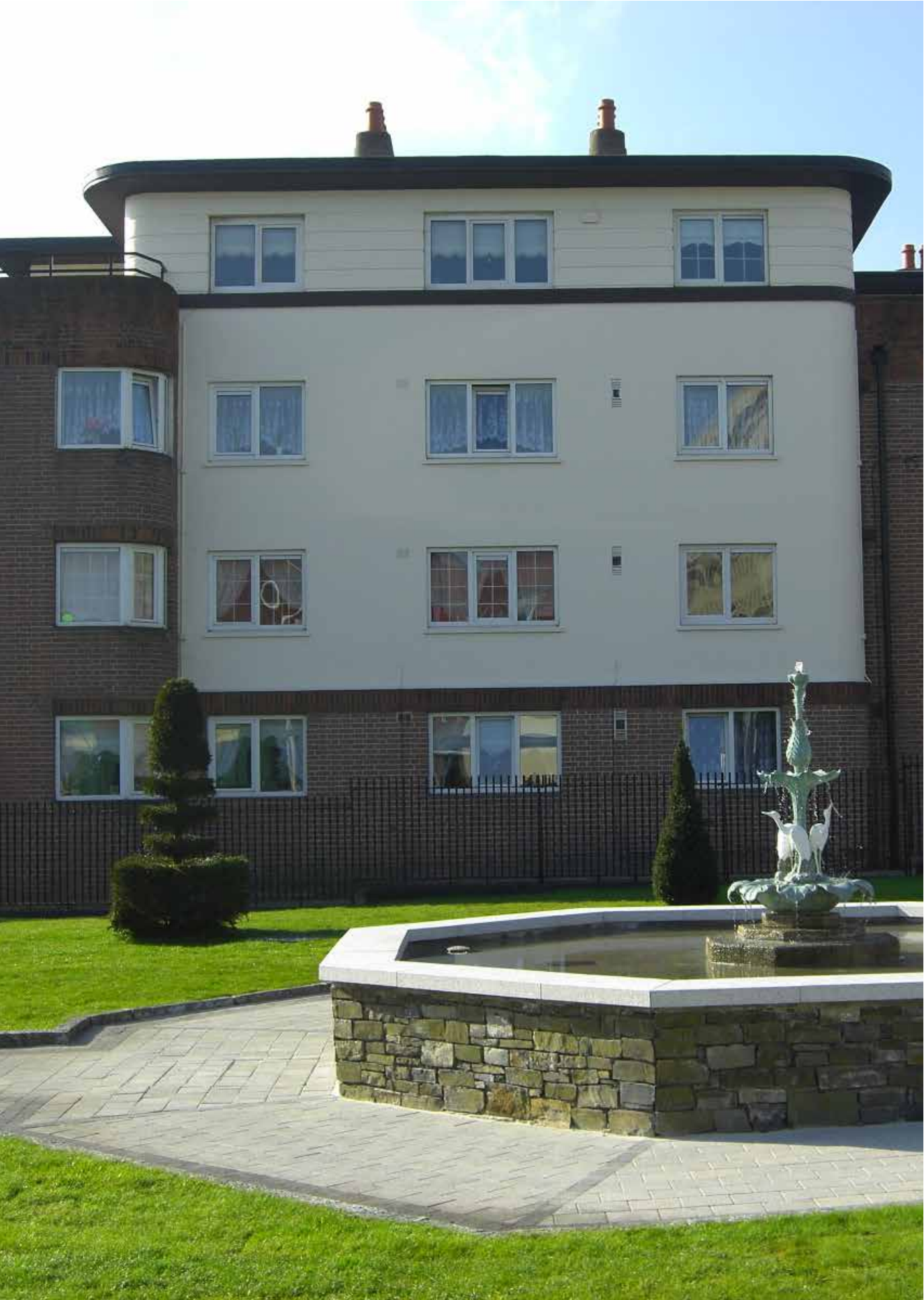
Chancery Street House and Chancery Park
